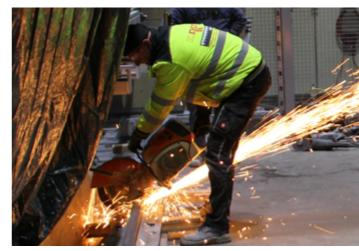
The worn racks were sawn up with the help of a cut-off grinder.
