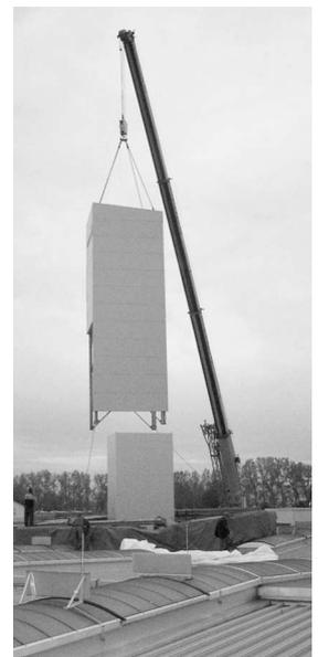
10 tonnes of steel were used in the new 12 meter high storage tower. The tailor-made steel outer covering protects the tower from wind and weather.
