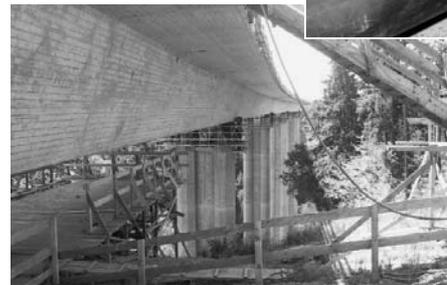
Under construction: Bridge made of pre-stressed concrete
