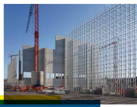
Impressive construction work in Nufringen: Before the side walls of the new logistics building extension are finally erected, by-passers are able to look inside the interior of the building. The high-rack shelving system is both a storage area as well as a load-bearing sub-structure for the roof and façade. Thanks to the compact silo construction, several thousand new storage spaces can be set up in the confined area. [JF]
