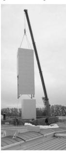
10 tonnes of steel were used in the new 12 meter high storage tower. The tailor-made steel outer covering protects the tower from wind and weather.
