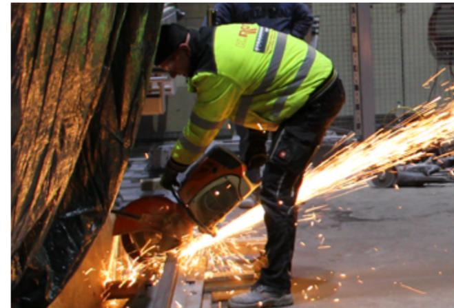
The worn racks were sawn up with the help of a cut-off grinder.
