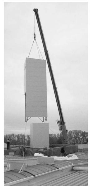
10 tonnes of steel were used in the new 12 meter high storage tower. The tailor-made steel outer covering protects the tower from wind and weather.
